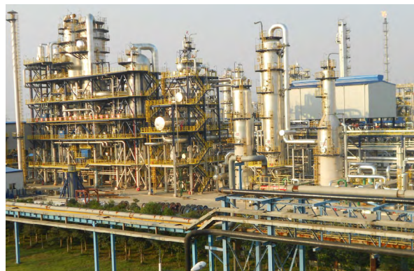
Operating MTO unit in Nanjing, China
