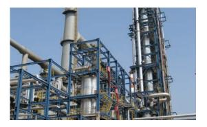
RecoveryMax is supplied as a modular system using proprietary equipment supplied by UOP. These include the UOP PSA system to purify hydrogen and the UOP PolySep<sup>™</sup> membrane to purify hydrocarbon from the PSA tailgas.
