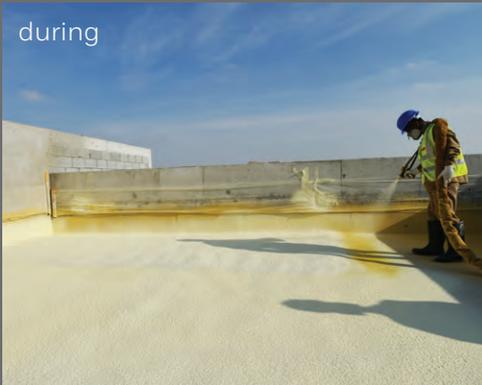
When applied, spray foam creates a seamless, monolithic insulation layer. There are no joints, fasteners and thermal bridges. It is water resistant, durable, and its strong adhesion properties help prevent roof uplift during high winds and extreme weather.
