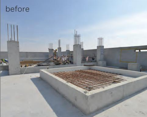
The spray foam system will insulate the concrete roof surface and provide a weather resistant seal around protrusions, parapets, and HVAC equipment.
