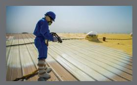
Spray foam was applied over the meta roof to prevent leakage and increase energy efficiency.
