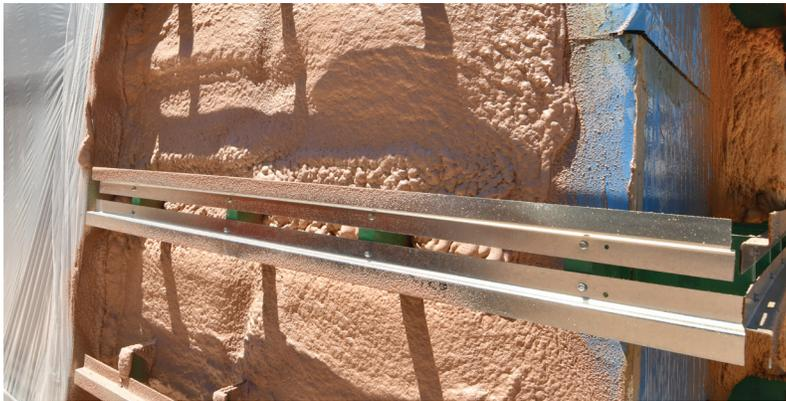
Insulthane Extreme featuring Solstice LBA was applied on the exterior walls to provide outstanding thermal performance and air tightness.
