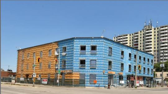
Closed-cell spray foam is being applied over the membrane on the exterior walls to meet Passive House requirements.
