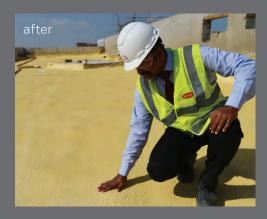
The foam is carefully checked after it hardens to ensure that the installation meets high quality standards.
