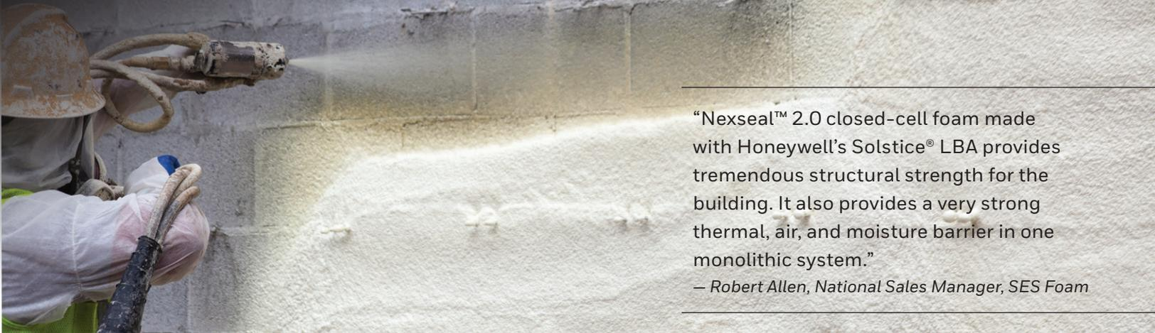
“Nexseal™ 2.0 closed-cell foam made with Honeywell’s Solstice® LBA provides tremendous structural strength for the building. It also provides a very strong thermal, air, and moisture barrier in one monolithic system.”
