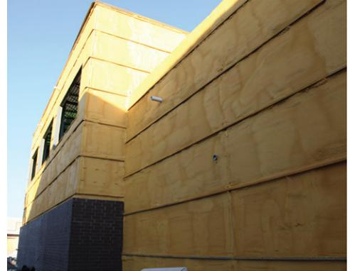
The closed-cell foam provided an all-in-one air, moisture, and thermal barrier while also increasing the building’s structural strength and durability.
