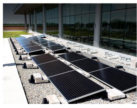
PV modules in a test installation from Tyll Solar in Rochester
